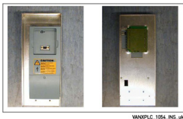
Figure 51. Control unit installed into the mounting box; Left: front; Right: back
